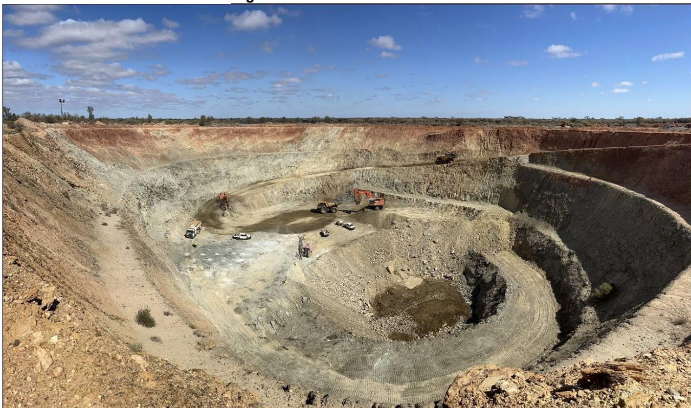
Figure 2.1 – Selkirk Cutback – end of October 2023
